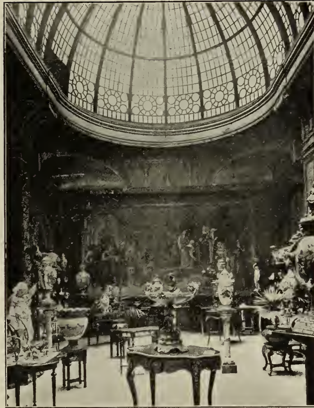
SKYLIGHT, COLUMBUS MEMORIAL BUILDING, CHICAGO.
